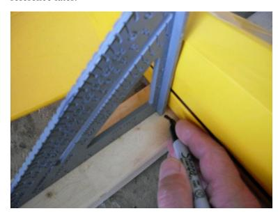
Using a square and the fuselage as a guide make two marks on the  $2\times3$  the width of the fuselage at the leading edge of horizontal stab. Each fuse will hang from its horizontal stab. The marks for the dowel holes need to be further apart than the width of the
