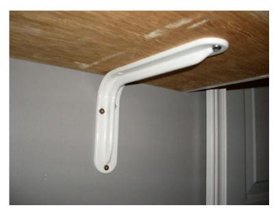
Using 2, 10in shelf brackets mount the shelf on wall, approximately 18in above floor ensure the area above the shelf is clear. I mounted mine a little higher to allow storage of the shop vac under it. Screw another 10-inch shelf bracket to the wall 30in above shelf aligned with left or right edge of shelf. Cut an 18-inch length of ½ dowel (or width of shelf used). Attach ½ dowel to upper bracket, cover dowel with pipe insulation. Place cup hooks at either end of dowel.
