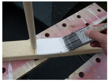
Prime and paint the wooden structure, I painted it to match the color of the wall. After the paint has dried it can be mounted on the wall. For typical drywall over stud construction walls use 4-inch (#10) wood screws or lag screws(with washer). In an earlier step you recorded the distance the  $2\times3$  was from the wall when the planes were arranged on the floor. Measure down from the ceiling this distance, this is where the hanger needs to be mounted.
